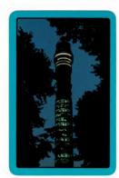
It was built by the Ministry of Public Buildings and Works 1961 – 1965 and weighs 13,000 tons. Its foundation, an 80 foot square and three foot thick pre-stressed concrete slab sits on the blue clay of London 22 feet below road level. Two high speed lifts carry visitors to three viewing platforms and the restaurant at, 1,000 feet per minute.
